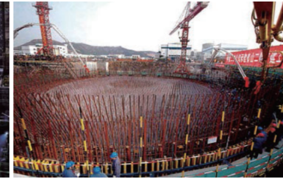
Qingshan Nuclear Power Plant Construction Site
