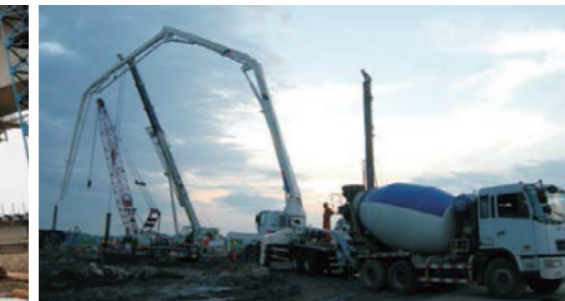
Hefei-Fuzhou CRH Construction Site
