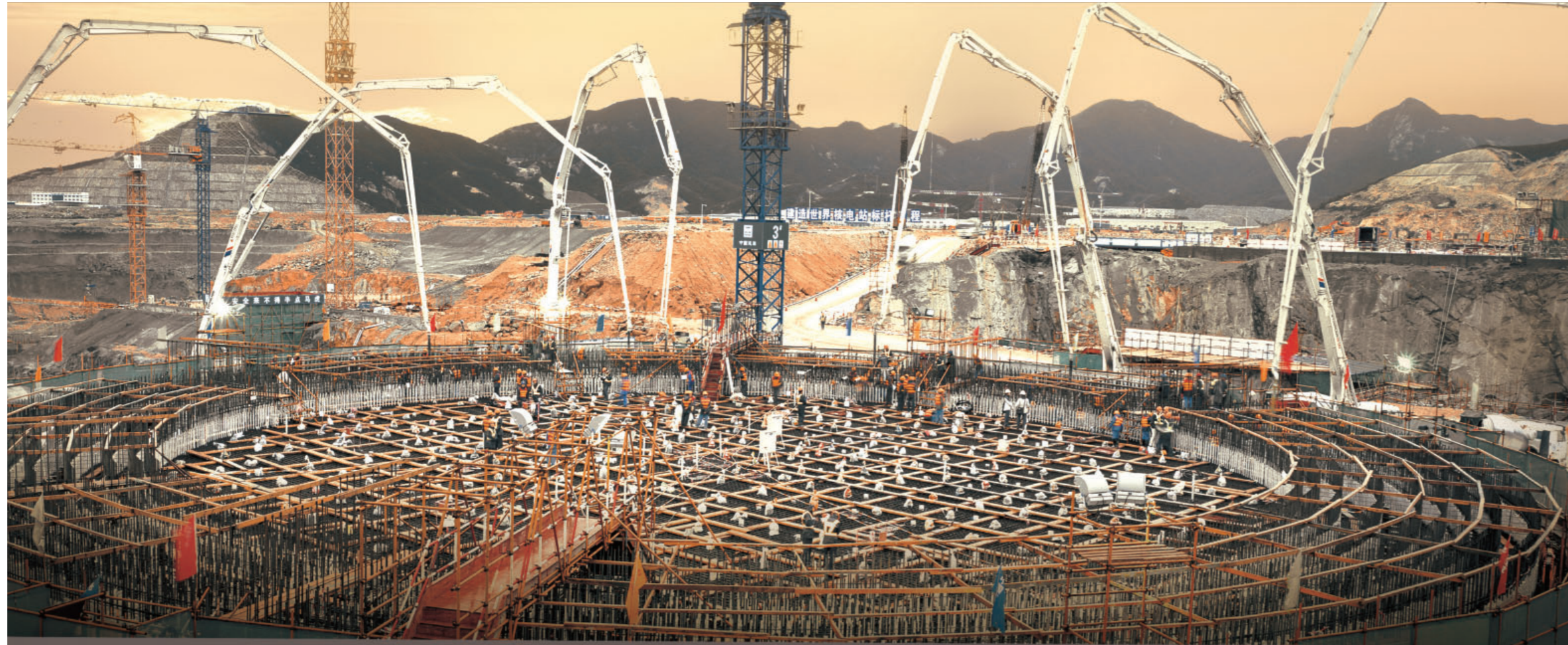
101 metres truck pump at Changsha Jiulonggang Construction site
