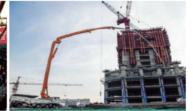
101 metre truck pump at Wuhanzhongxin Construction site
