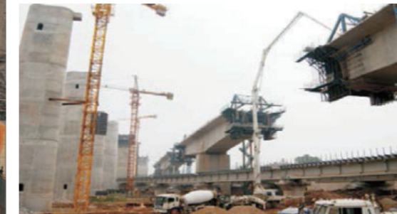
Shanghai-Jiangsu CRH Construction Site
