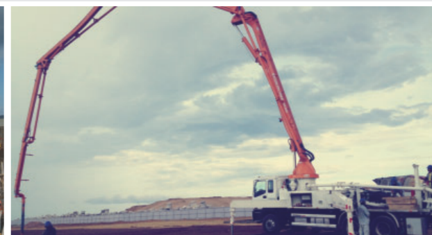
FPC steel mill project, Ky Anh, Vietnam
