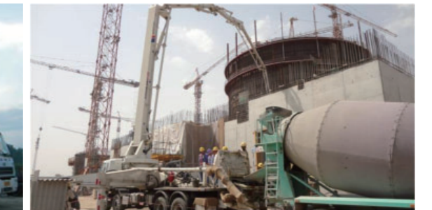
Nuclear Power Plant C3 Project, Pakistan
