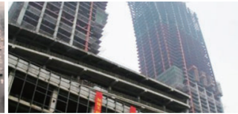
Gate of the Orient, Suzhou Construction Site
