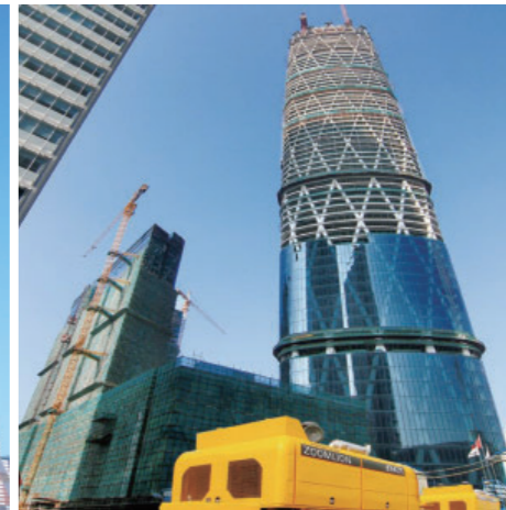
Construction Site of West Tower of Zhujiang New City, Guangzhou
