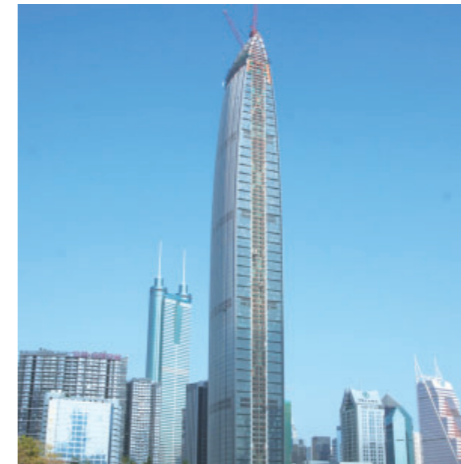
Kingkey Financial Center Construction Site, Shenzhen
